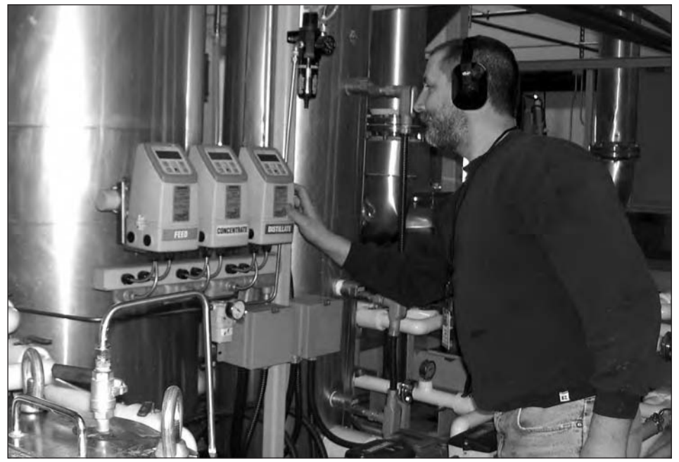
A technician runs a system check on Inland's Glycol Concentrator at Bradley. This patented system uses about one-tenth the energy of traditional distillation systems to separate water from the waste chemical.
