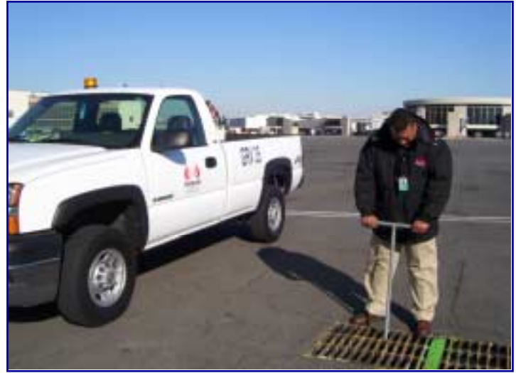
Rob Alvarez, Inland's Site Supervisor at Washington's Reagan Airport, uses a T-bar handle to open the GlycolGuard™ drain. The drains are closed prior to de-icing taking place and opened once weather permits.
